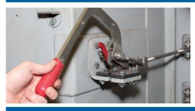
The locking trigger secures the door clamp during operation. Easy to follow instructions are provided for installing replacement triggers. New clamp assemblies are also available.
