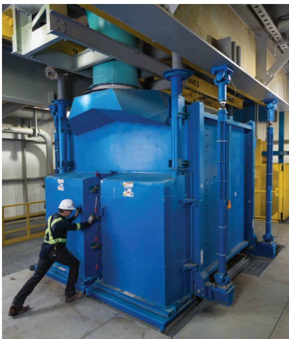
Figure 4: Rotex minerals separator Model MM5430-1-S, Bethune installation
