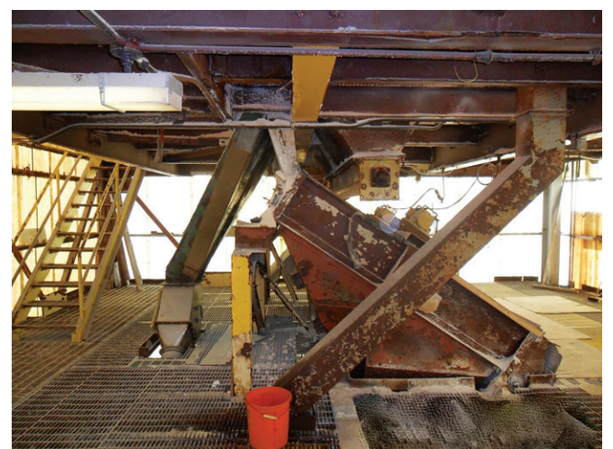
Figure 1: Original installation of high incline vibratory screeners and chute work
